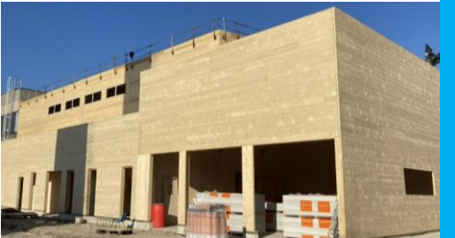
New Thermal Treatment project in Amiens
