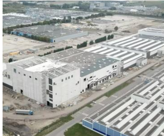
Location of the future Gigafactory in Douvrain (France)
