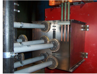
Fig. 2. Vertical Electrode configuration
